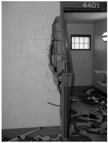
Segregation Unit: Concrete block walls destroyed by weight bars
