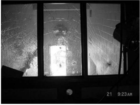
Housing Unit Control Center: Windows broken by inmates throwing projectiles
