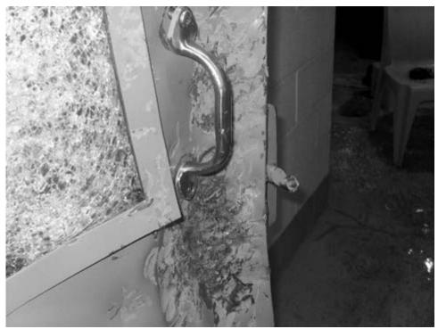
Housing Unit Control Center: Inmates used weights to break windows and destroy locking mechanisms to access control centers and electronic panels.
