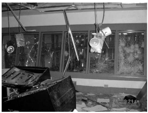
Housing Unit Control Center: Inmates gained access and damaged sprinkler systems, control panel and windows overlooking unit.
