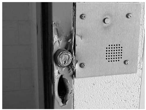
Locking mechanism destroyed by weight bar
