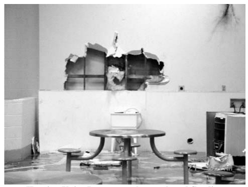
Housing Unit: Damage to sheetrock and flooding
