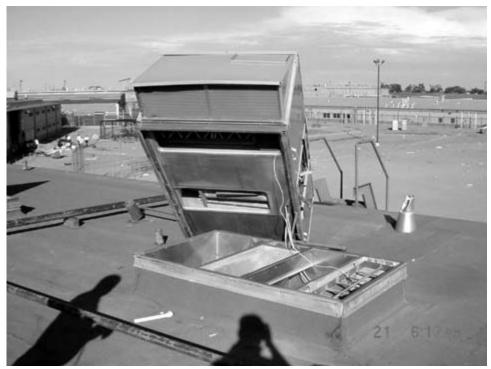
Unit 1: Inmates damaged air handling units after accessing roof through escape hatch, above control center.
