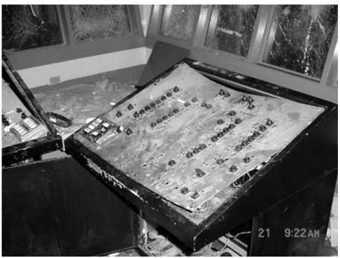
**Housing Unit Control Center: Electronic panel destroyed**
