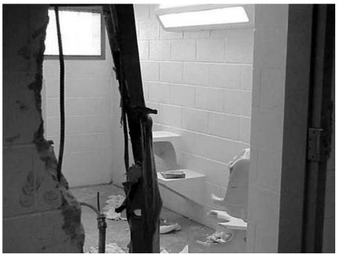
Segregation Unit: Cell door compromised, porcelain fixtures destroyed; flooding
