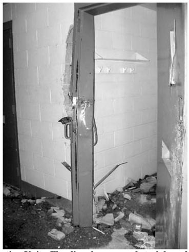
Segregation Unit: Flooding damage and steel door defeated
