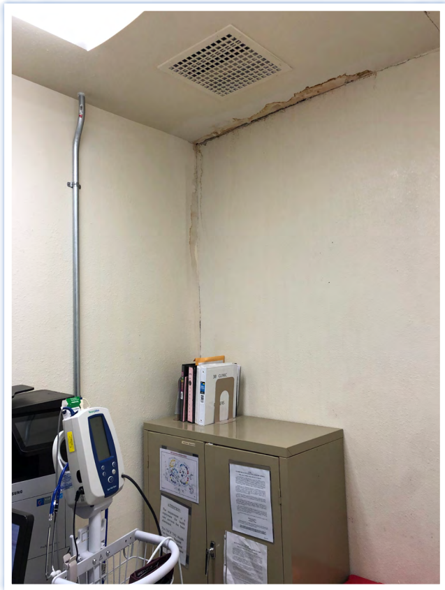
Photos 4, above, and 5, right. Residual water damage (photographed on March 12, 2020).
