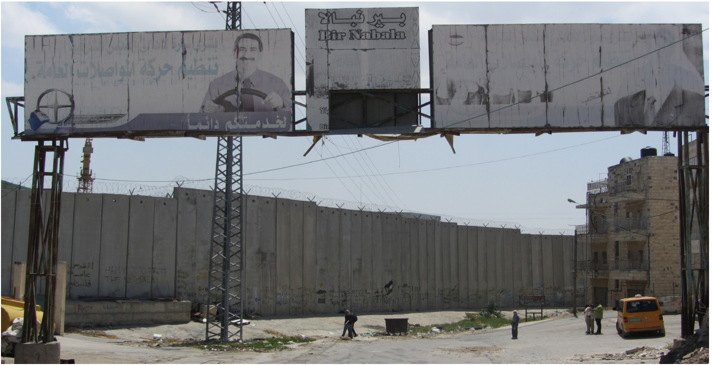
Former main street of Bir Nabala, now cut off by the Wall, making it a ghost town.
