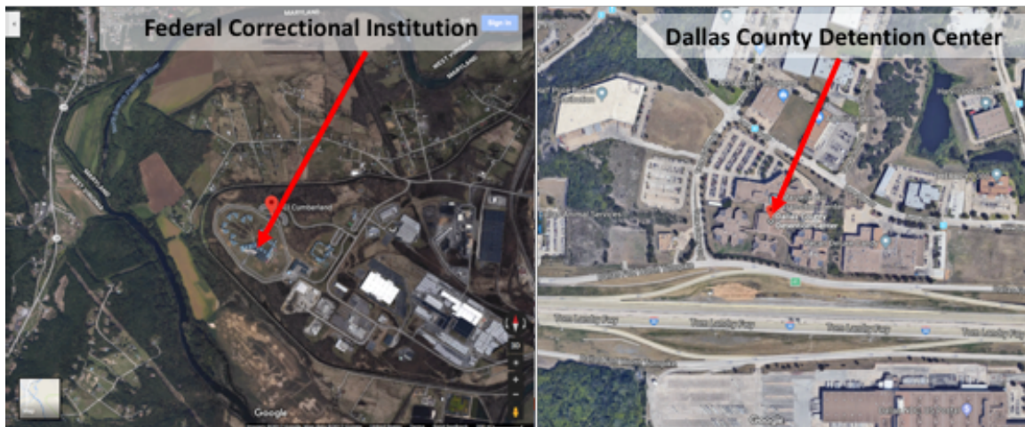
Figure 1. Federal Correctional Institution (Left) and Dallas County Detention Center (Right)
