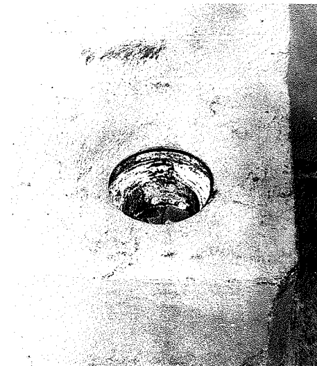
The "Chinese toilet" or hole in the floor in a Draper doghouse cell.
