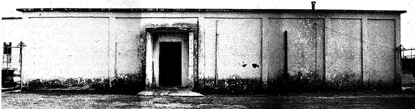
The infamous "doghouse" at Draper Correctional Center in Alabama. "This windowless concrete building and the cells in it had no lights, no ventilation, no toilets, no furniture, no beds, no running water, and no sinks or showers."
