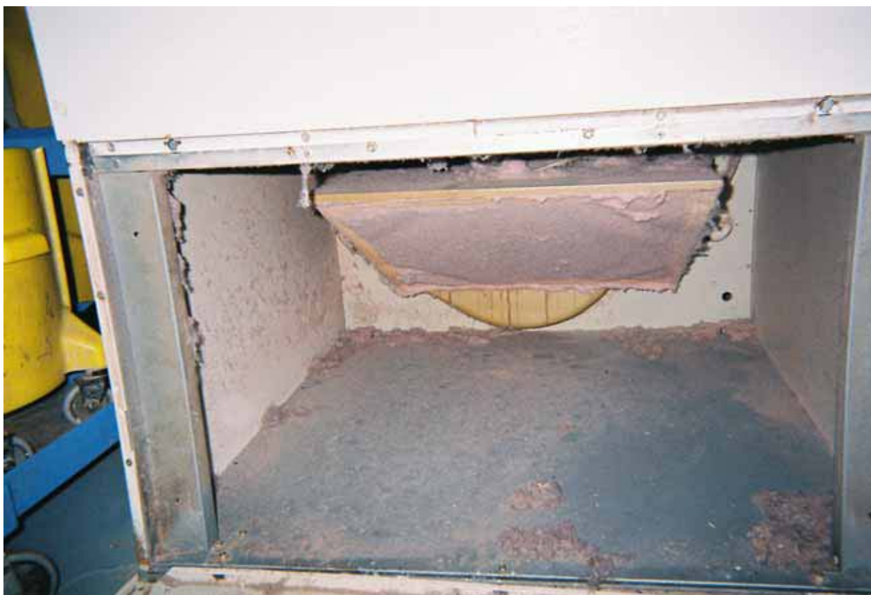
Clogged lint-trap under the only operational dryer on campus (for nearly 200 youth) creating another fire hazard
